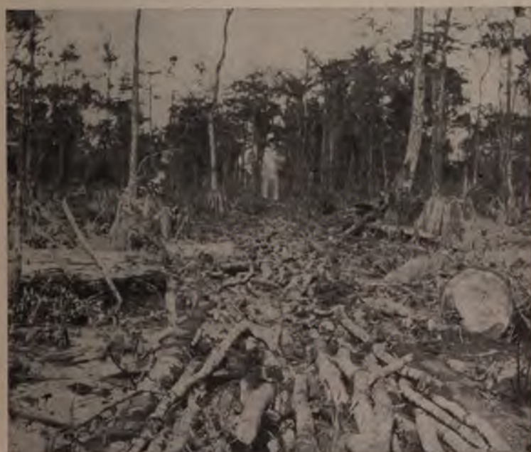
FIG. 79.— The Foundation for a Dunnage Road. Louisiana.
